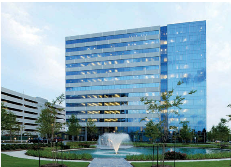
Dallas-based Trammell Crow Co. and Des Moines, Iowa-based Principal Real Estate Investors have received LEED Silver certification for Energy Center I, a 332,000-square-foot (30,840-sq-m) office building located in Houston and fully occupied by Foster Wheeler USA.
